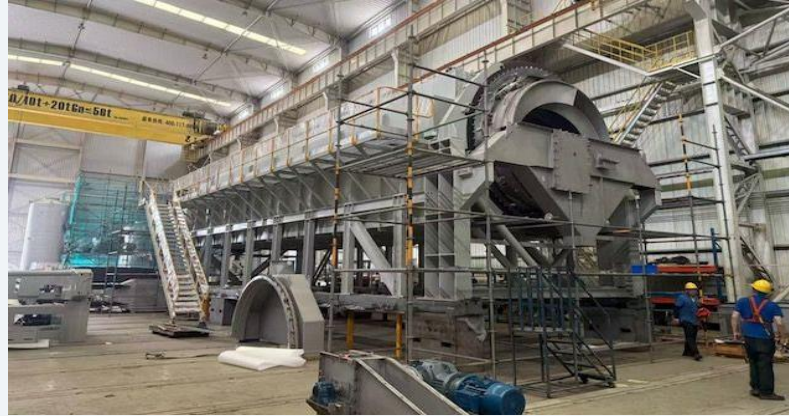
Calcliner trial assembly completed
