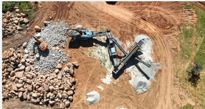
Aggregate plant commissioned
