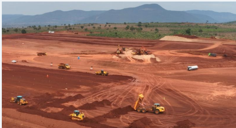
TSF boxcut underway
