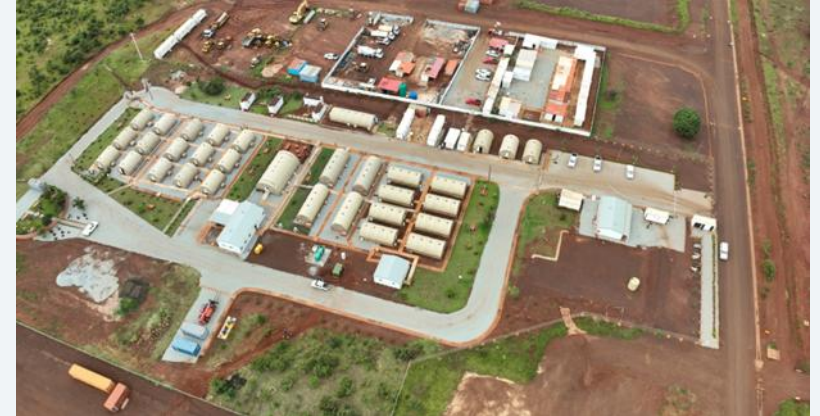
Construction camp completed
