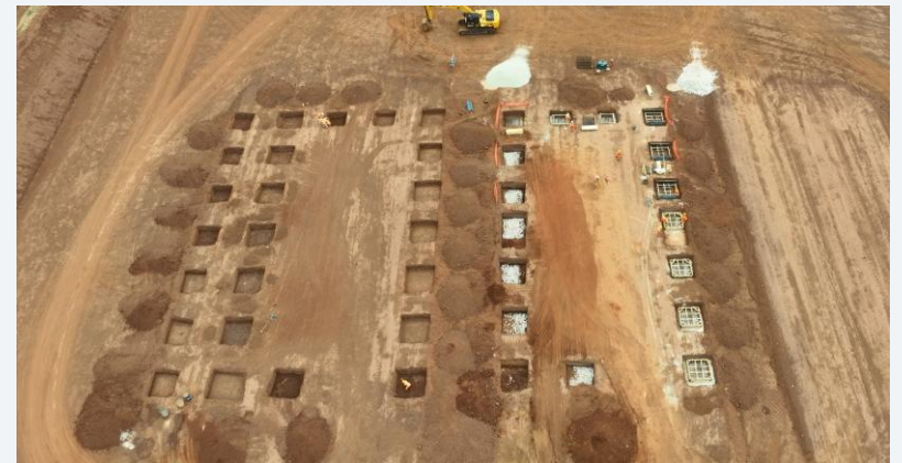
Bulk earthworks undertaken
