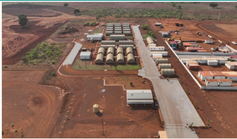
350 Person camp installed
