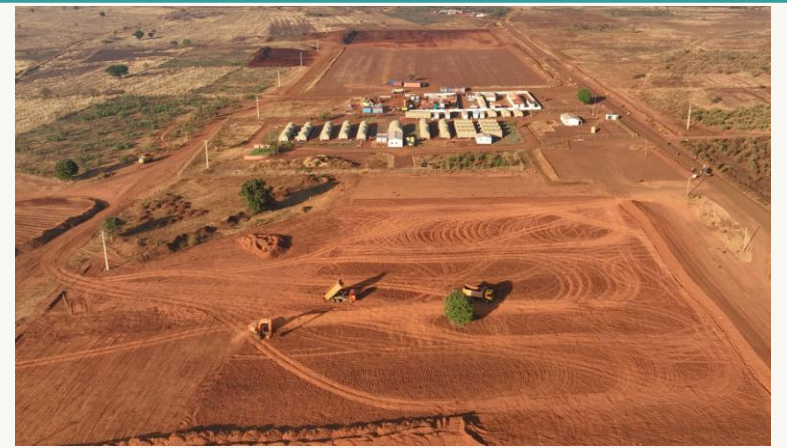
Contractor laydown area
