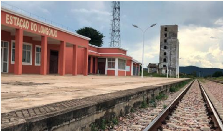
Longonjo railway station - 4 km from mine
