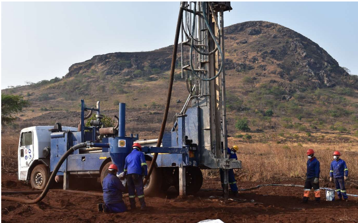
Drilling commences at the Longonjo NdPr Project.
